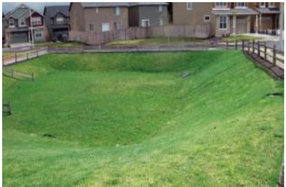
Detention Pond (Dry Pond)
