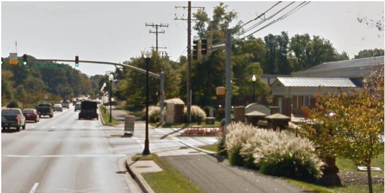
3. Shared Use Path Along Forest Drive
